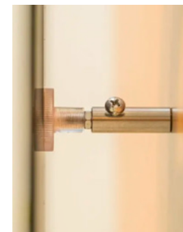
Distance holder secured to the wall and attached to the glass
